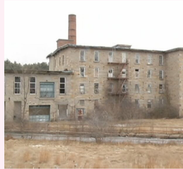
Hope Village Cotton Mill in Hope, RI. I spent two weeks during my thesis fall housesitting in this tiny town within Scituate. Formerly one of the largest textiles mills in the nation now lies in disrepair and abandon multimedia
