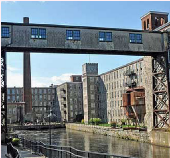
Royal Mills, West Warwick, RI, Exterior view, looking west down the Pawtuxet River, South branch.
