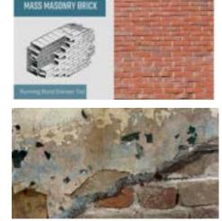
This page, top right: Typical Mass Masonry Brick Construction. Source: International Union of Bricklayers and Allied Craftsmen
