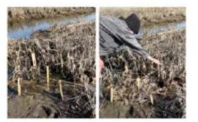
The second prototype was crafted using rectangular wooden stakes intertwined with natural fibers, forming a sturdy net structure. Additionally, fallen marsh grasses were integrated into the weave to bolster its resilience and act as a barrier against incoming tides, facilitating sediment accumulation.
