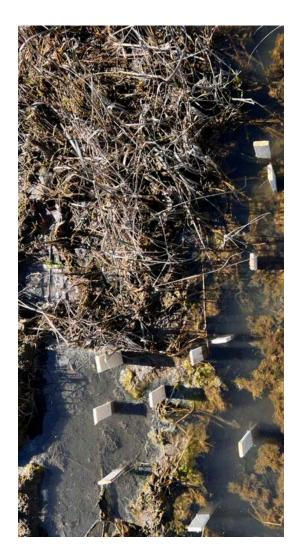
The third prototype was erected along the same canal but positioned farther away from the main channel, where water flow is notably gentler. It was constructed using rectangular wooden stakes arranged to create a three-dimensional grid structure, strategically designed to trap sediments gradually. Notably, this prototype drew upon insights gleaned from the prior iterations, particularly regarding the timing of construction (during the lowest tide) and site selection.
