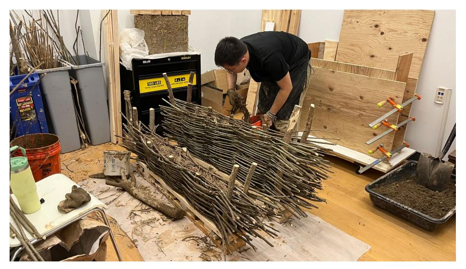
After the building process, the Streamco willow whips start to take root and germinate, which proves the possibility of the straw clay in wattle frames to be a living and evolving system.
